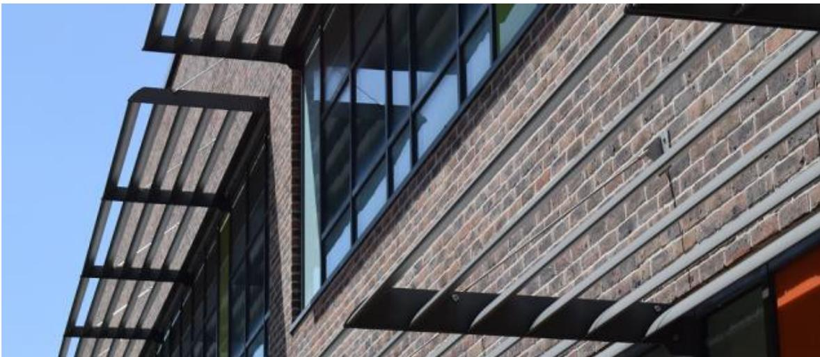
Image 20: Solar shading above windows at Southmead Hospital Pathology Building
